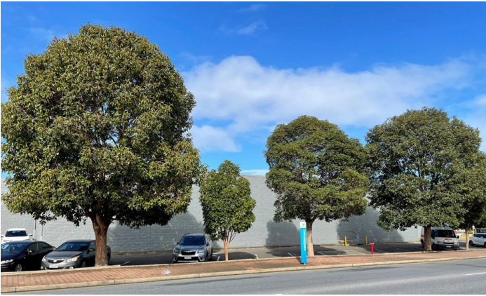
Castle Plaza Shopping Centre wall for mural, Raglan Avenue, Edwardstown
